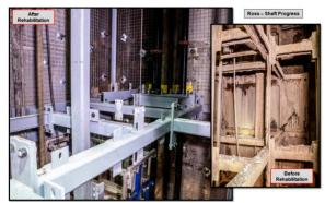
Figure 5: Ross Shaft – before and after steel removal
